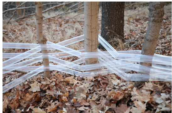
Fig. 1: Example shelter wall composed of inflated tubes interleaved between existing environmental features.
